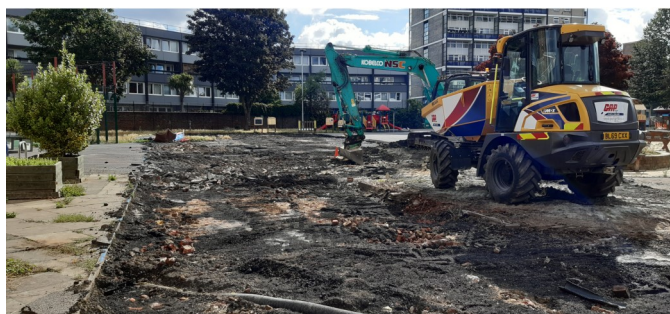
Site clearance works
