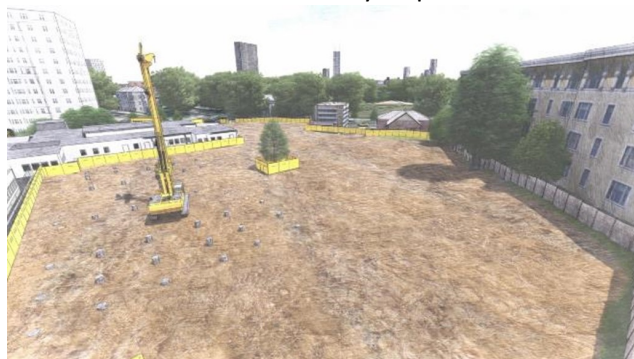
Early Site Works
